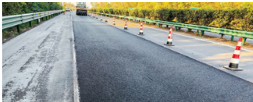
Applying steel slag asphalt concrete technology for expressway pavement maintenance
